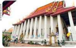
Phra Ubosot Built during the reign of Rama I, the imposing boht (ordination hall) as it stands today is the result of renovations dating back to the reign of Rama III (r.1824–51).
