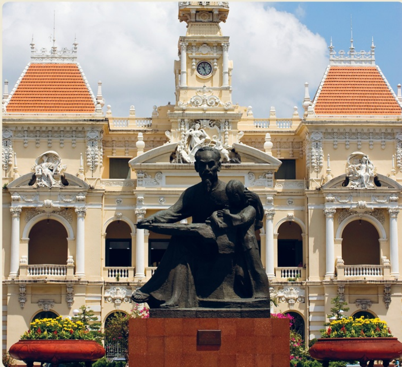
City Hall building, Ho Chi Minh City
